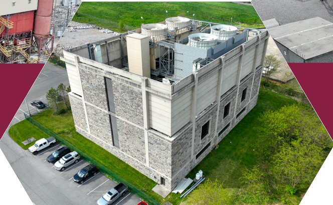
Chilled Water Plant
